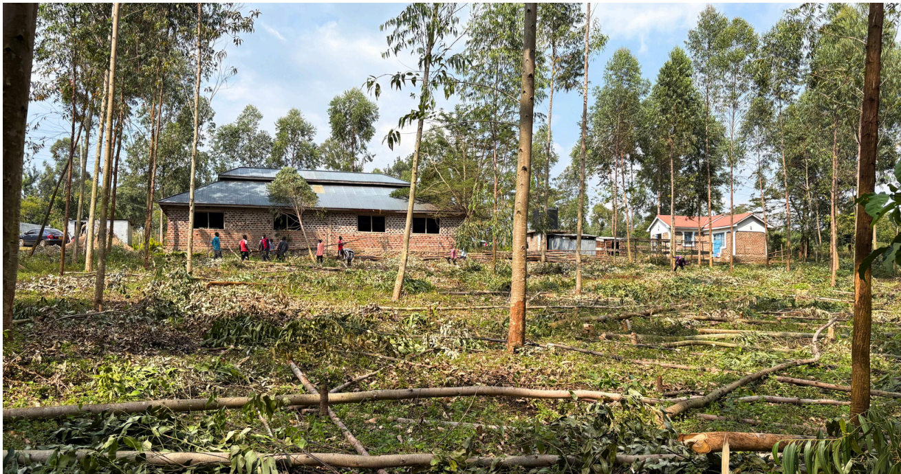
The previous barn structure with the water tower and caretaker's house to the right.
